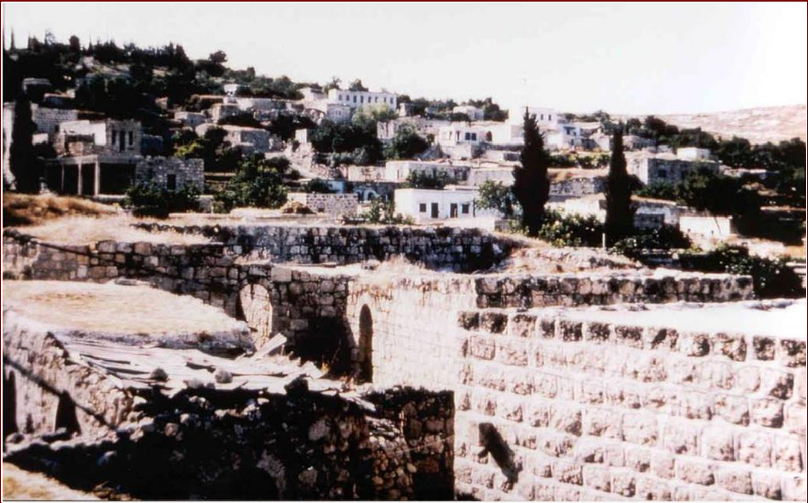
21. The village of Emmaus, Ramle Sub-District, was completely erased from the map in 1967. All homes and buildings, the Catholic Church, a Convent, and two Muslim Mosques were razed and 5,000 Arabs made homeless in Emmaus and the neighboring Arab villages of Beit Nuba and Yalu.
