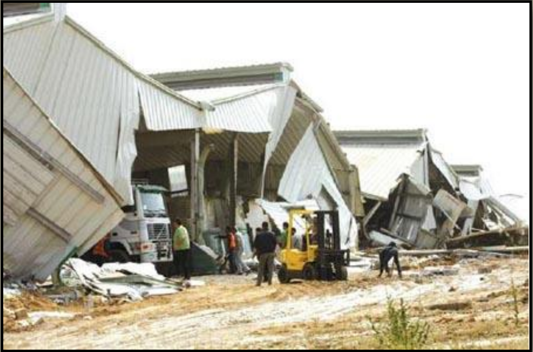
Even after «Cast lead» the destructions continues: 21 april 2011
