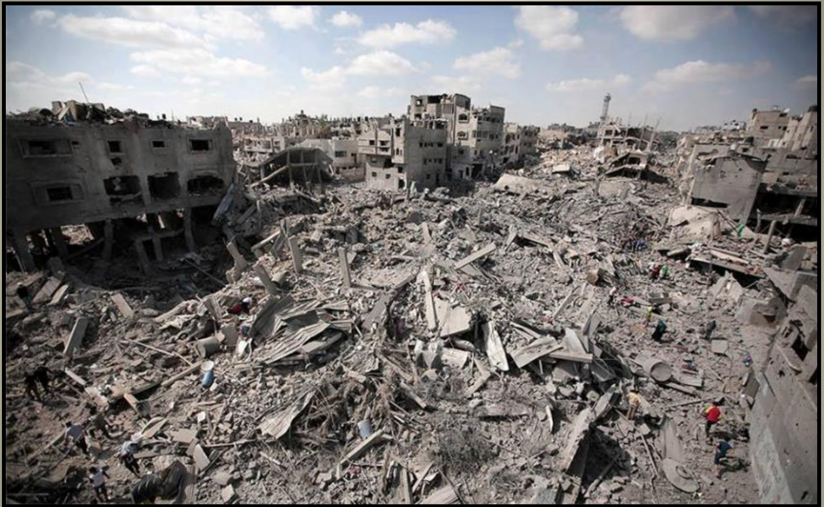
AFTER - Gaza, July 2014: note the extent of destruction
