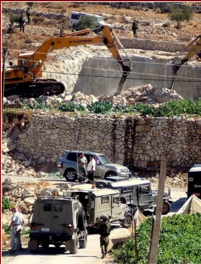
Demolition of an underground water tank 03.09.2009
