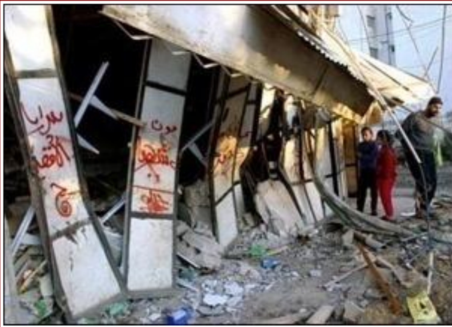
Destroyed shops in Gaza
