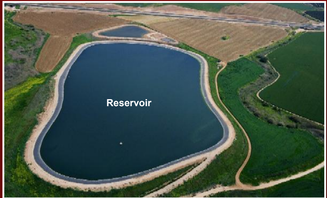
Sea water desalination
