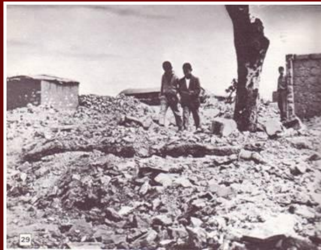
Destruction of the camp of Jabalia
