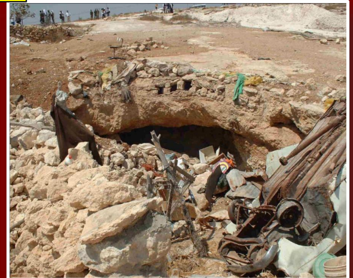
In Susiya this cave was also destroyed , it was being used as a home by a poor Palestinian family. Why?
