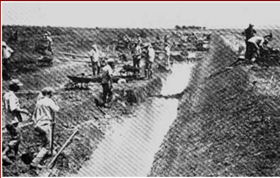
Beginning of the 1920s: drainage construction
