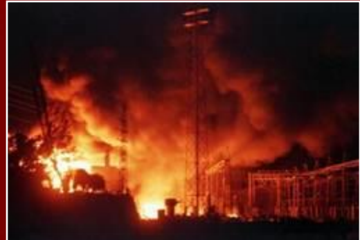
The power plant of Joumhour destroyed by the Israelis on 8.2.2000
