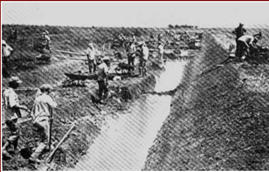
Beginning of the 1920s: drainage construction
