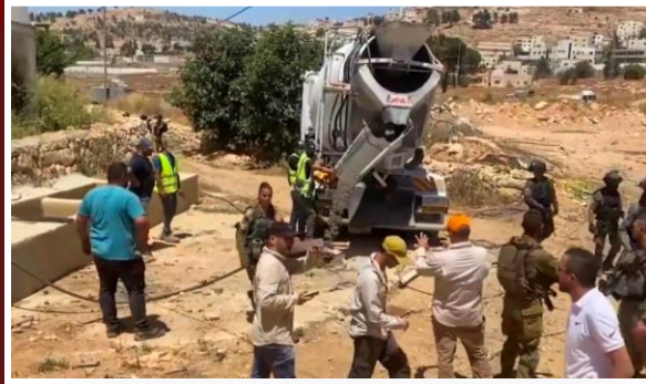
Cementation of a well, Hebron, 7.27.23
