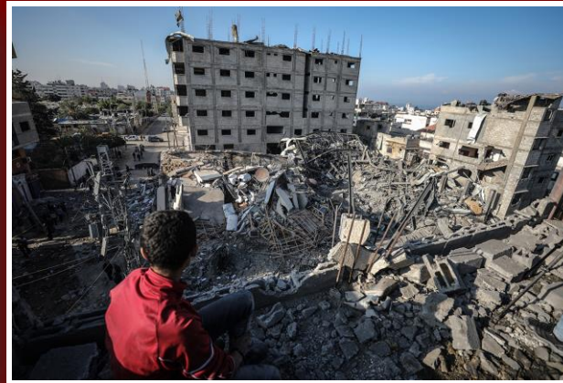
The rubble of al-Alqsa TV studios Gaza 12 November 2018
