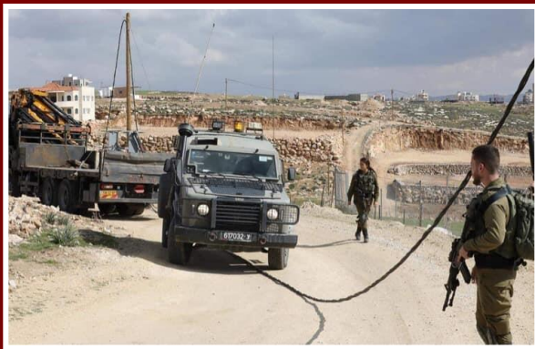
Electrical and telephone lines
