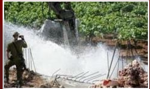
Demolition of the water-reservoir of a Palestinian farm
