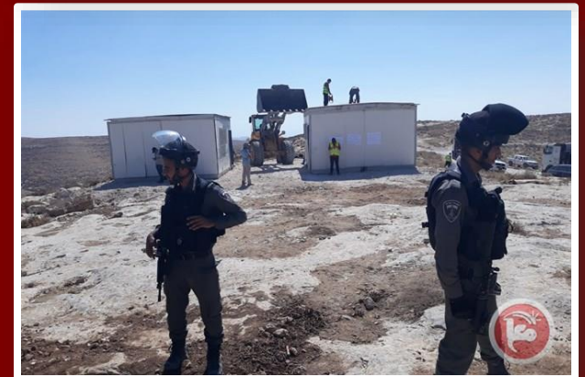
School demolition and removal in at-Tuwani village, southern Cisjordan. July 11, 2018
