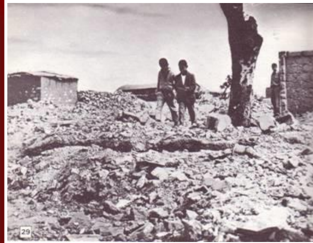
Destruction of the camp of Jabalia
