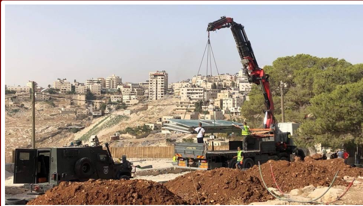
Demolition of the kindergarten at Jabal al-Baba, East Jerusalem July 25, 2018
