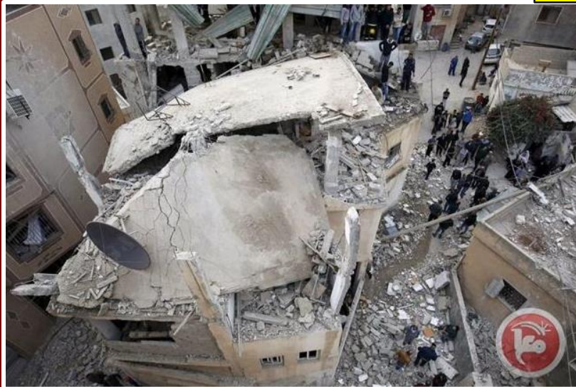
Qalandiya refugee camp, 16 November 2015. House destroyed because two Palestinians suspected of killing an Israeli settler lived there. Two Palestinians were killed on site, 17 were injured. (Maan)
