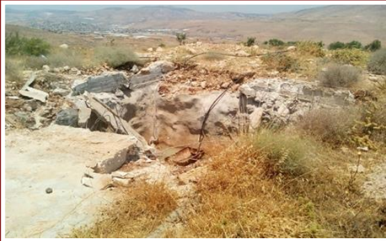
Demolished water well in Um Kbeish. The Israelis also demolished Palestinian houses and uprooted olive trees. June 11, 2019.
