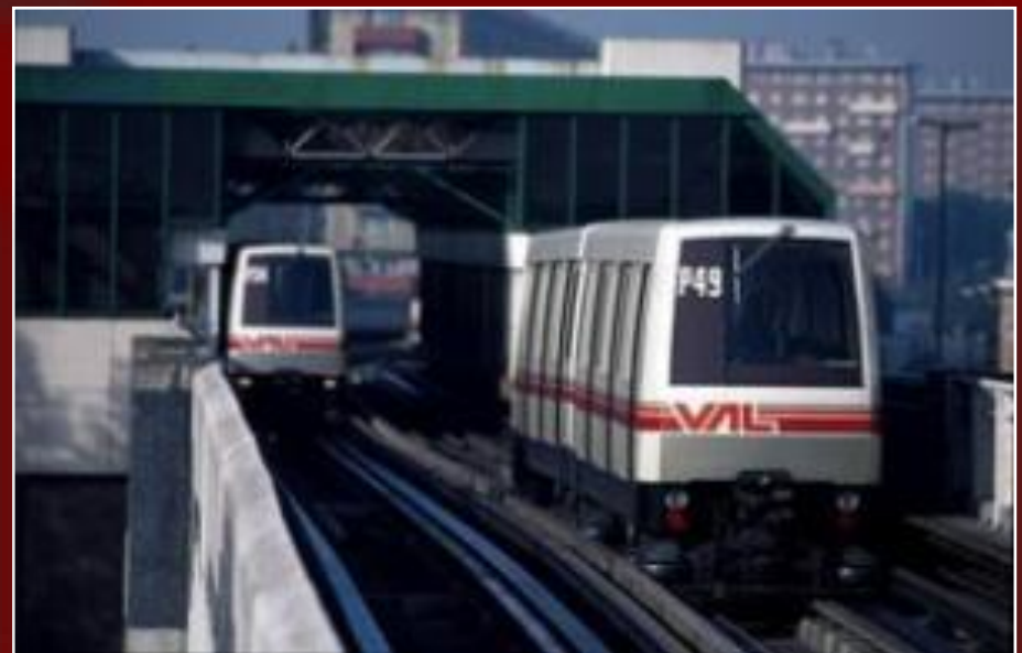
Lille: automatic underground
